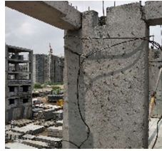
Figure 16. Notch connection
