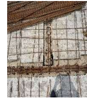
Figure 18. Beam to beam connection
