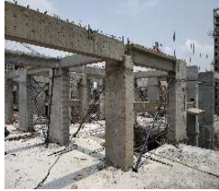
Figure 15. Beam resting over column
