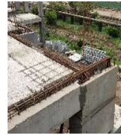
Figure 17. Column to beam connection
