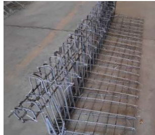
Figure 2. Beam Reinforcement
